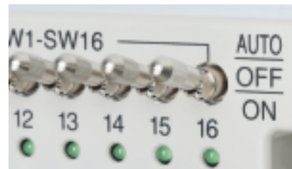
Hold toggle switch installed
